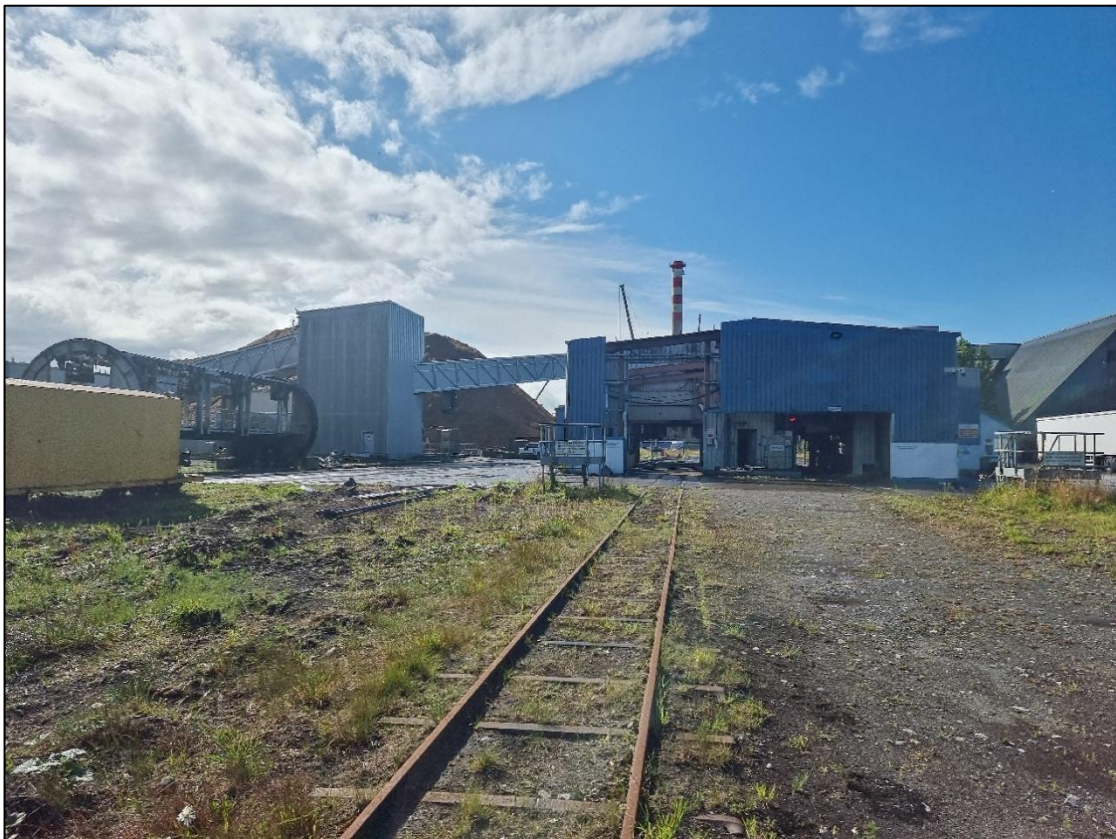
Plate 4-31 Edenderry Power Station (background) in the west of the site is classified as Buildings and artificial surfaces (BL3).
